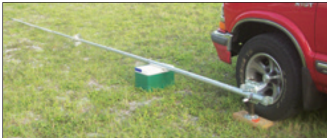
Figure 4 — The mast is in place ready to be elevated with the help of the jack.
