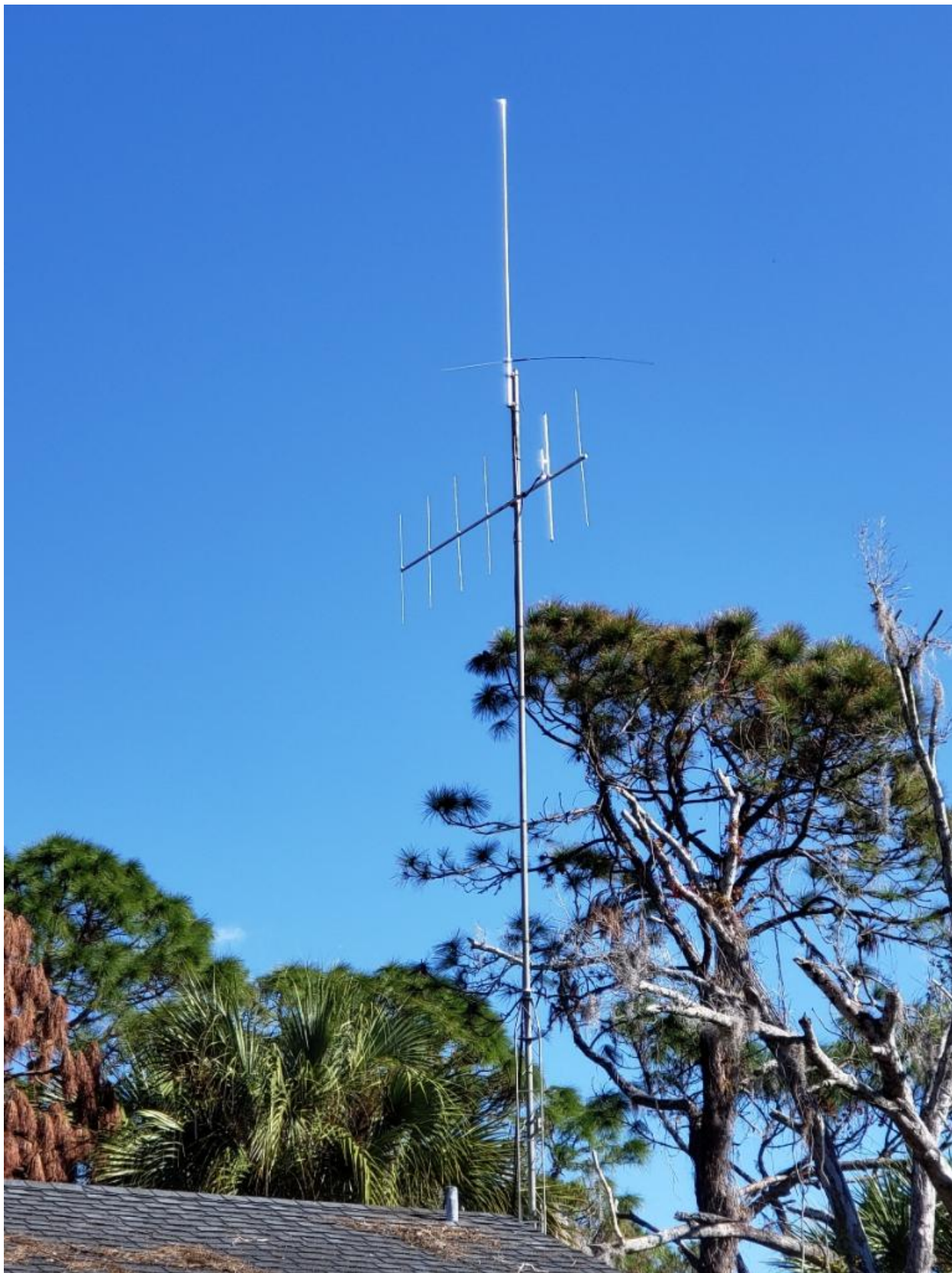
Here's a picture of Tony's rebuilt antenna "farm!" Very nice!!
